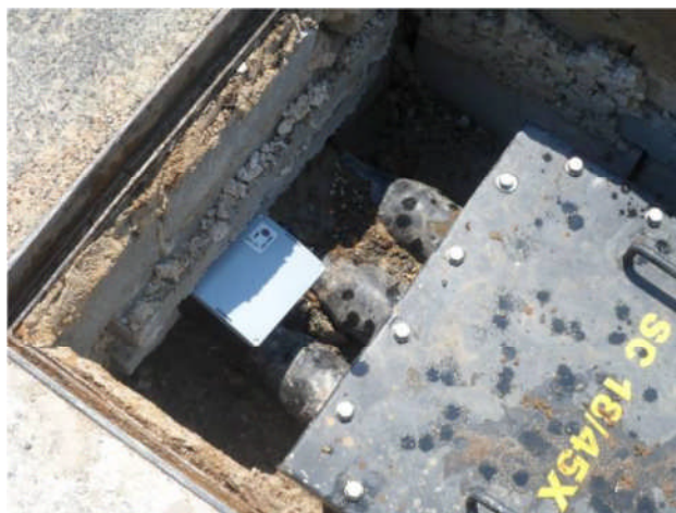
Example of measurement on a cable joint (screen earth near linkbox).
