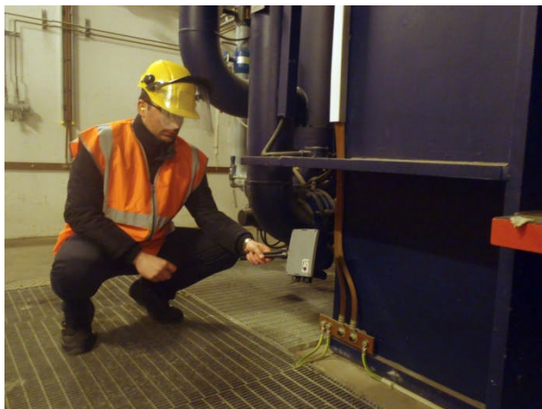
Example of measurement on a power transformer (transformer earth).
